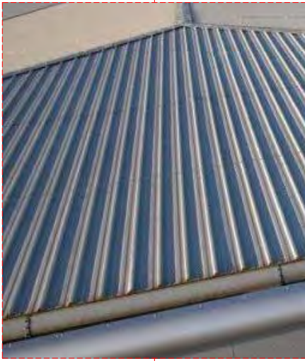
Kingspan Roof Span Finish : Surf Mist Description : Pre-finished insulated trapezoidal sheets on suitable support framing, forming a metal deck roof covering.
