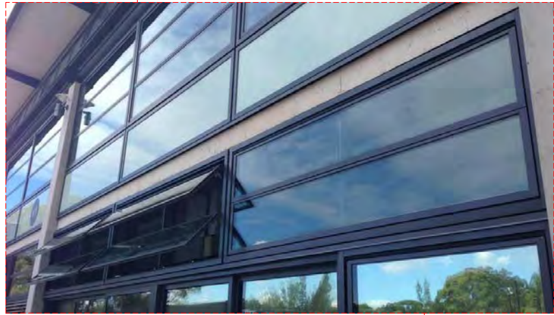
Framed Mechanical Louvres Finish : White powdercoat Description : Operable louvers to provide natural ventilation.
